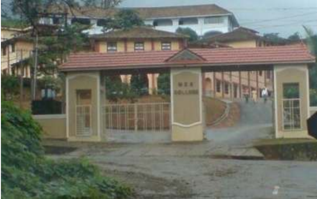
Figure 1 MAIN ENTRANCE OF COLLEGE
